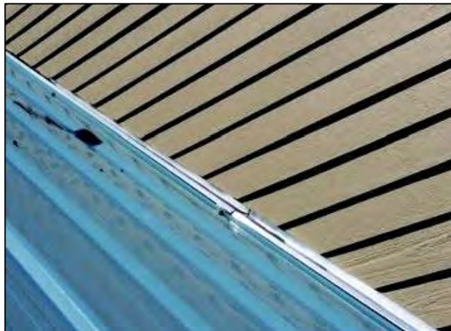
Figure 9 - Flashing at New Building Facade Installed Incorrectly
