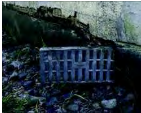
Figure 8 - Crawlspace Vent
