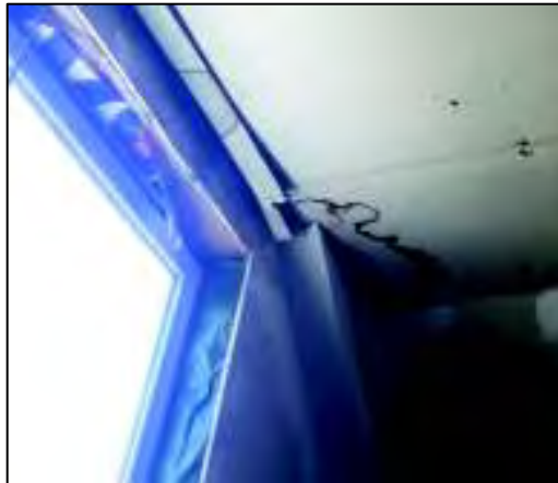
Figure 20 - Dry Moisture Stain on Ceiling
