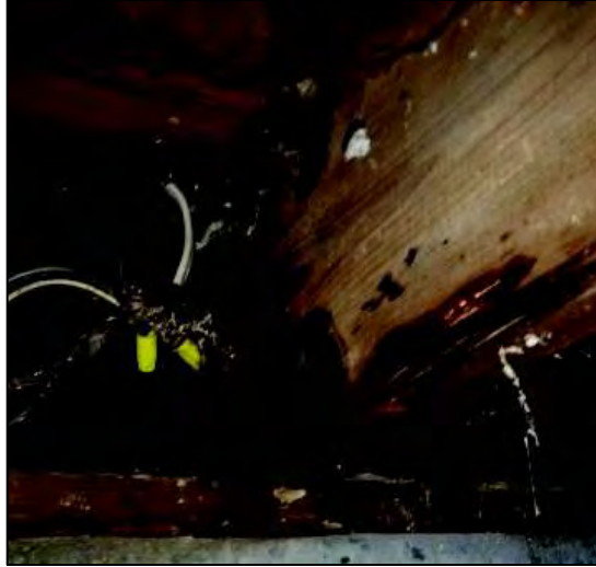
Figure 7 – Moisture Damage in Crawlspace and Electrical
