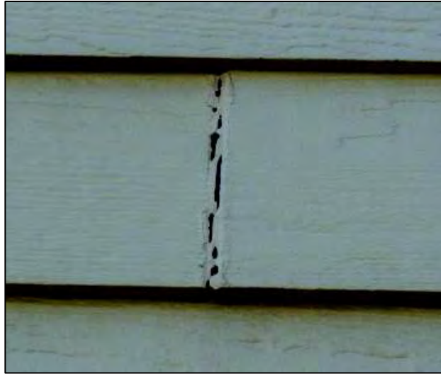
Figure 13 - Hardie Plank Siding Separating @ Joints
