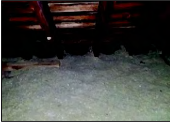
Figure 24 - Insulation Covering Overhangs in Main Hall Roof
