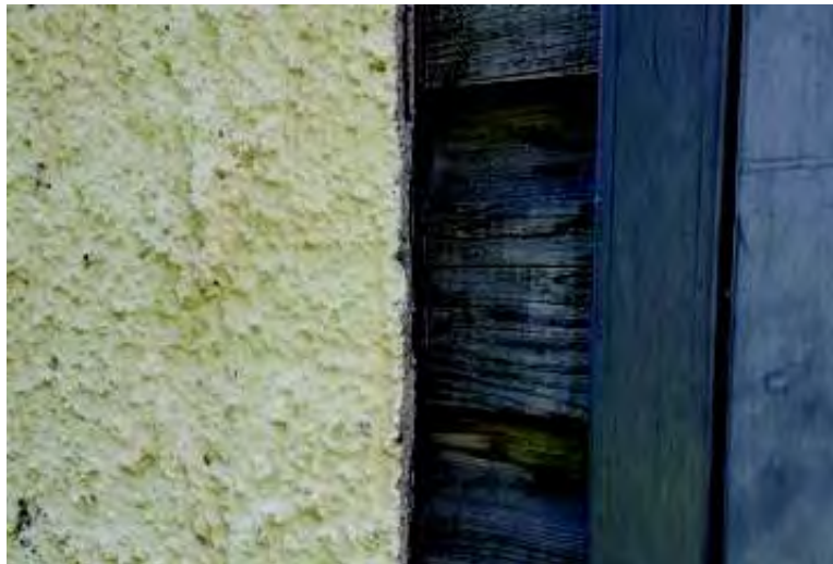
Figure 12 - Stucco Over Original Wood Siding
