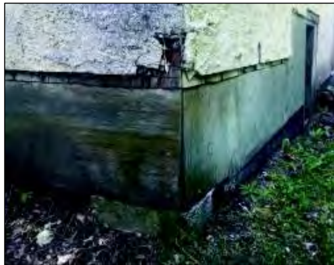
Figure 5 - North East Corner Sill Plate (Dry Rot)
