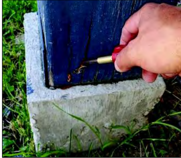
Figure 17 - Dry Rot @ Balcony Post
