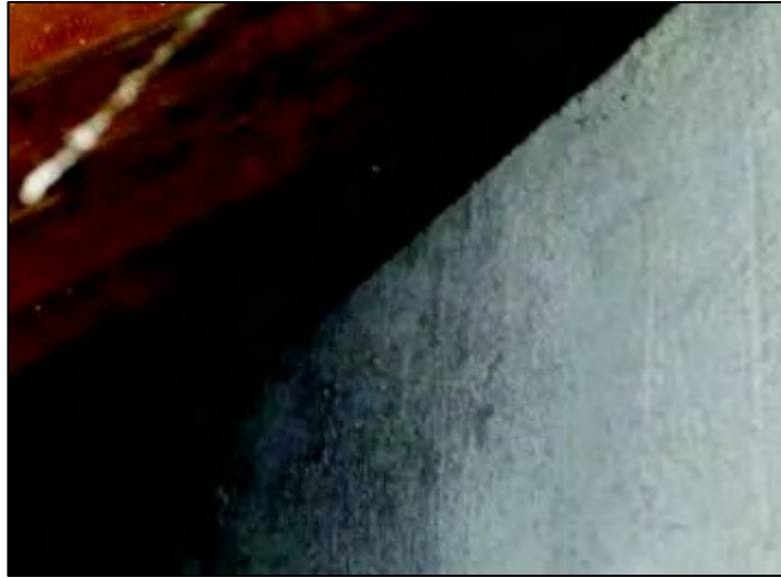
Figure 3 - No Ledger Board @ Kitchen Rafters
