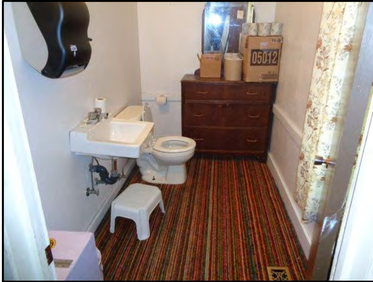
Figure 12 - Carpeted Bathroom with Poor Ventilation
