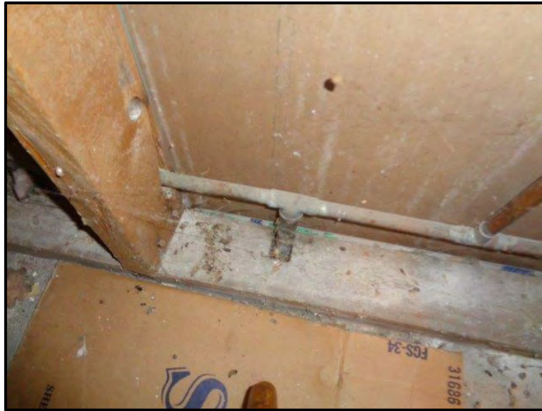
Figure 14 - Water Service Pipe
