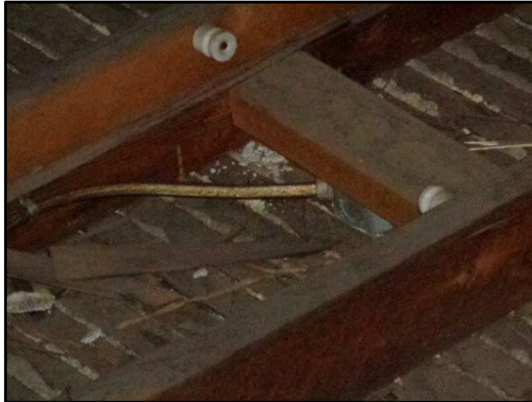
Figure 13 - Disconnected Electrical in Attic
