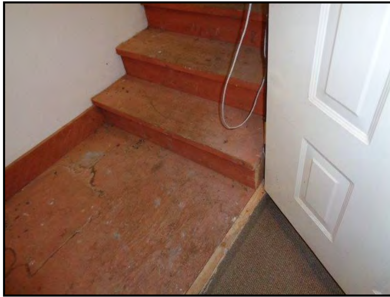
Figure 3 - Evidence of Moisture in Basement Stairwell
