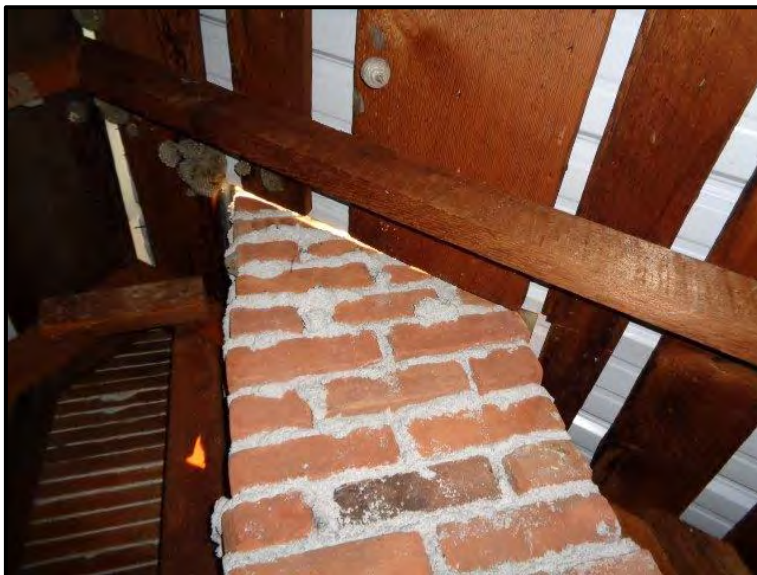
Figure 5 - Poor Flashing and Weather Sealing of Chimney
