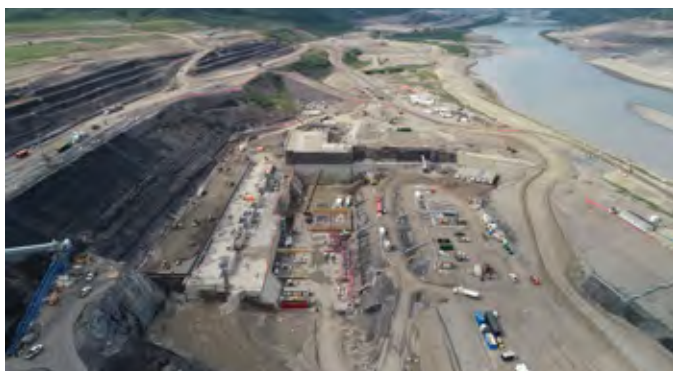
The Site C powerhouse buttress and main service bay pad, looking upstream, in August 2018.
