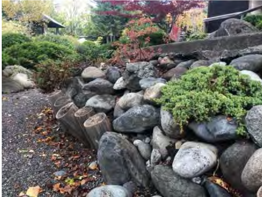
Failing Cedar Posts and Slumping Rock Wall in Present Garden
