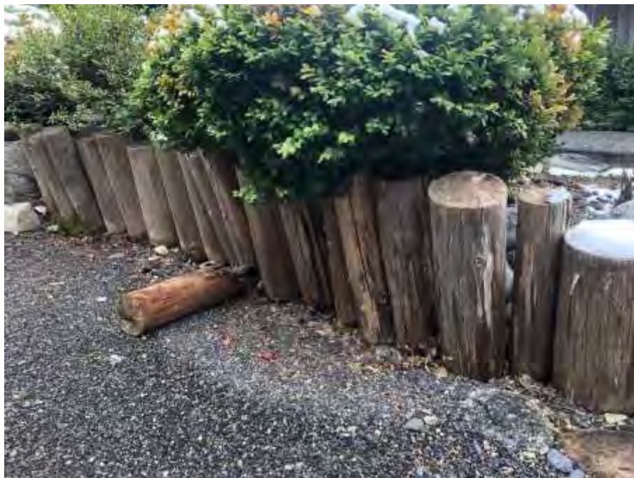
Failing Cedar Post Retaining Wall with Visible Rot in Future Garden
