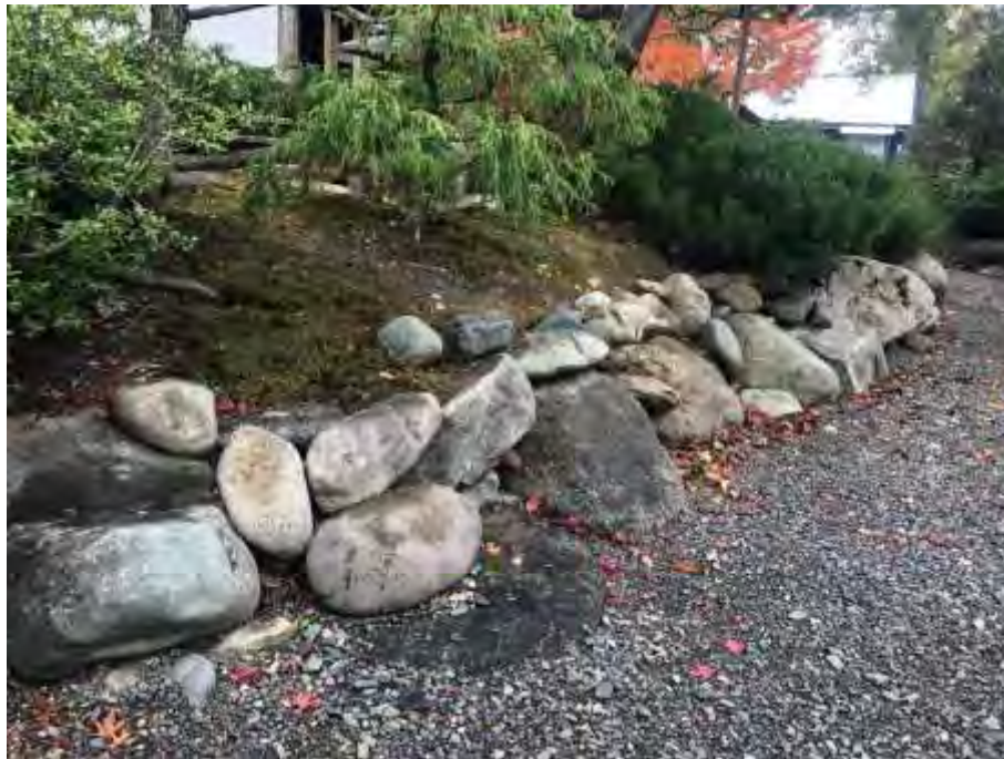
Slumping Rock Wall in Present Garden
