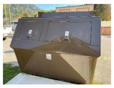
Ten 4-cubic-yard refuse containers are provided by the Village for use by commercial properties. These are emptied twice a week by staff. The entire container is hydraulically lifted and dumped into the collection truck.
