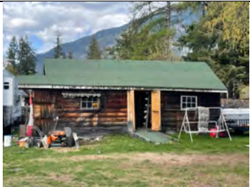
28x14’ modified as shed. 6-pane sliding windows. Original style roofing & shiplap siding exposed (Hut #200, 2nd Ave.)
