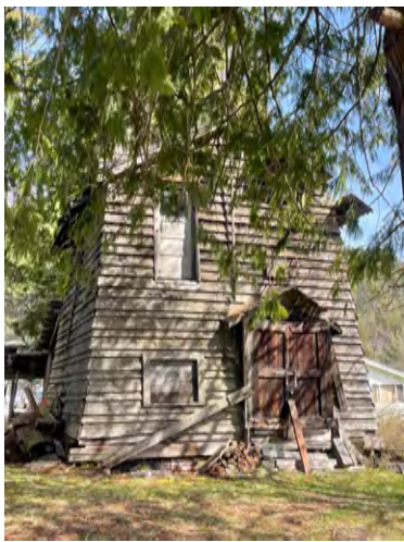
The original camp water tower, now a storage shed. Posts through the roof supported the water tank, and water was piped to hydrants around the camp for firefighting. An original hose reel lies behind the hatch left of the doors. (1st Ave.)
