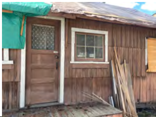
28x14’ modified as shed. 6-pane sliding windows. Original style roofing & shiplap siding exposed (Hut #200, 2nd Ave.)
