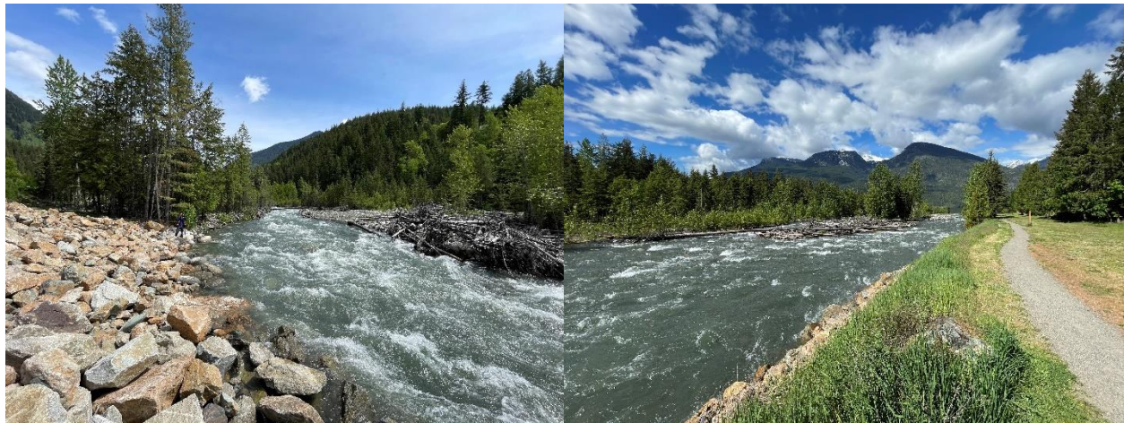
Photo 6: Upstream view of large wood jam opposite the recently repaired section of dike upstream of the Bridge (left) and downstream view of mid-channel jam downstream of the Bridge that is bifurcating flow (right).
