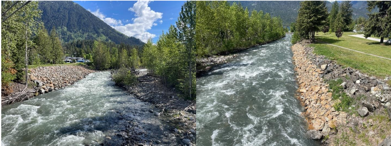
Photo 7: Recently placed rip-rap following scour during the 2020 flood (orangey tan colour). Rip-rap repaired upstream of the bridge (left, upstream view) has larger material (up to 1,200 mm), whereas the downstream portion (right, downstream view) has smaller material (up to 400 mm). The smaller material has a higher chance to be displaced based on the sediment mobility analysis.
