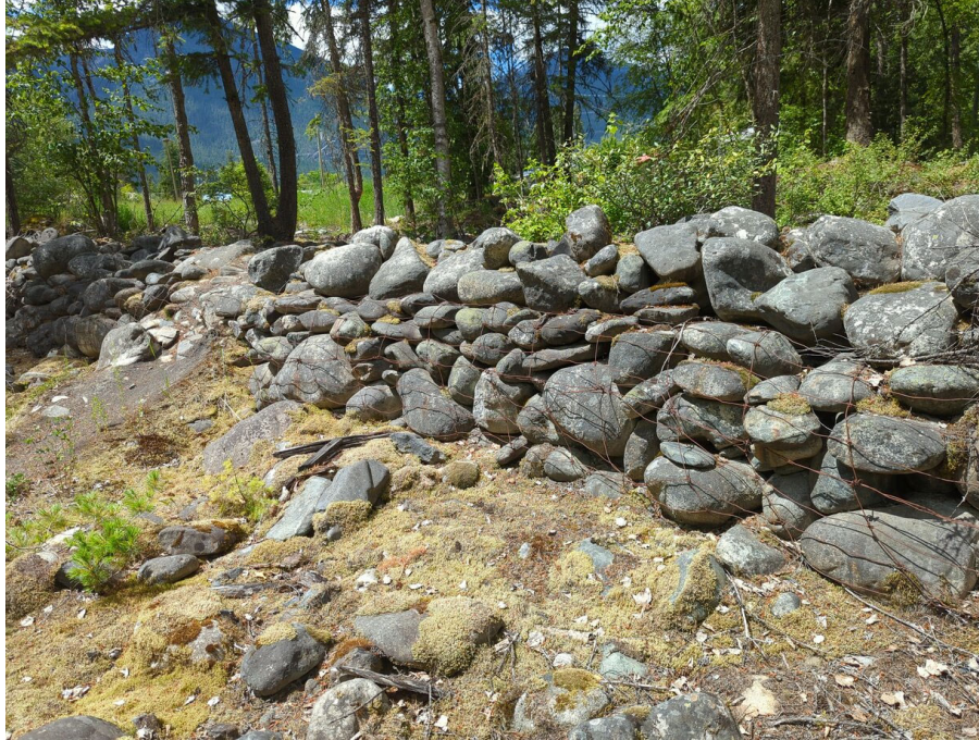
FIGURE 2-4: RELIC BANK PROTECTION CONSISTING OF ROCK WRAPPED IN WIRE
