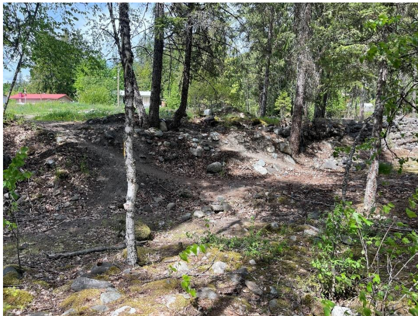
Photo 8: Northeast view along the upstream portion of the dike protecting the Bridge, looking toward the intersection of Slocan Avenue and Columbia Street. Note this section of dike, although locally set back from the active channel, is constructed of erodible, cobbly fan deposits.
