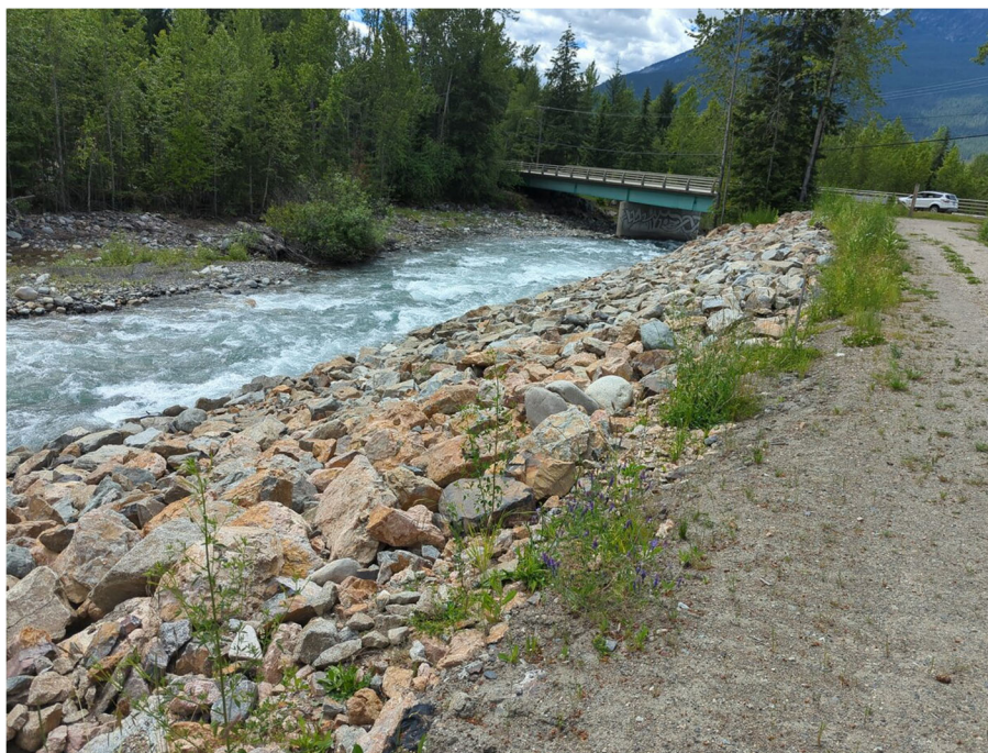
FIGURE 2-2: EXISTING RIPRAP PROTECTION UPSTREAM OF HIGHWAY 6
