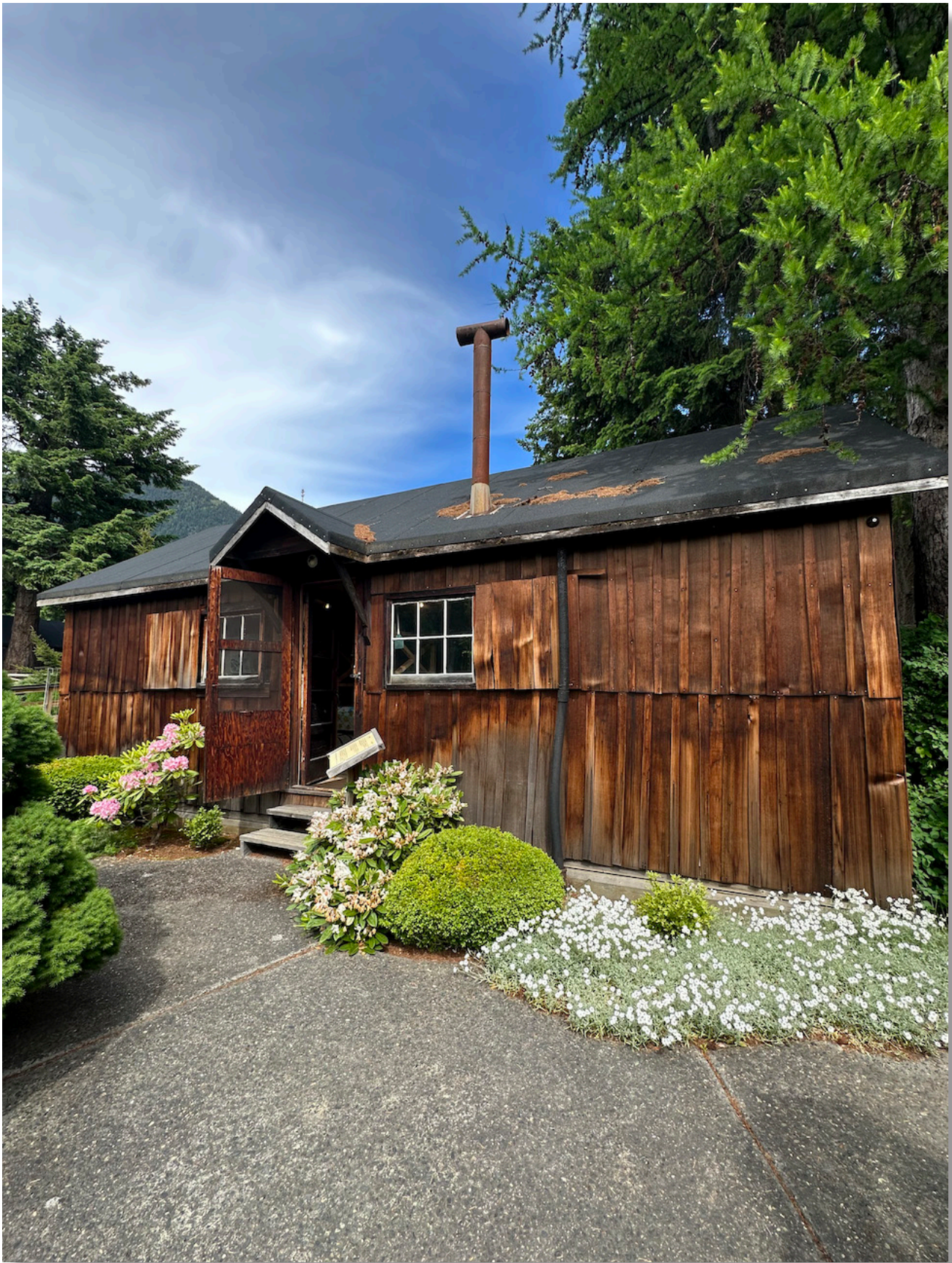
Exterior view of internment shack at NIMC. Courtesy of the NIMC.
