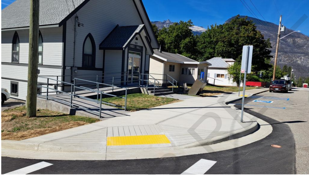
Outdoor accessibility improvements at Knox Hall.
