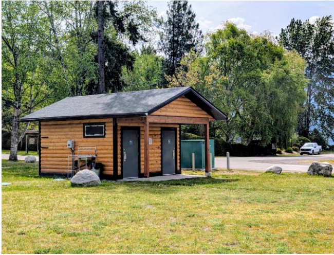
New public washroom at Centennial Park.
