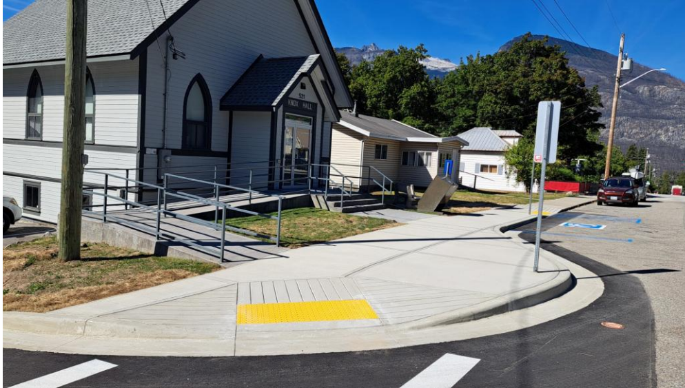
Outdoor accessibility improvements at Knox Hall.
