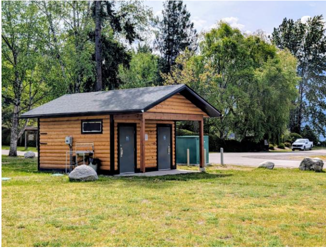
New public washroom at Centennial Park.
